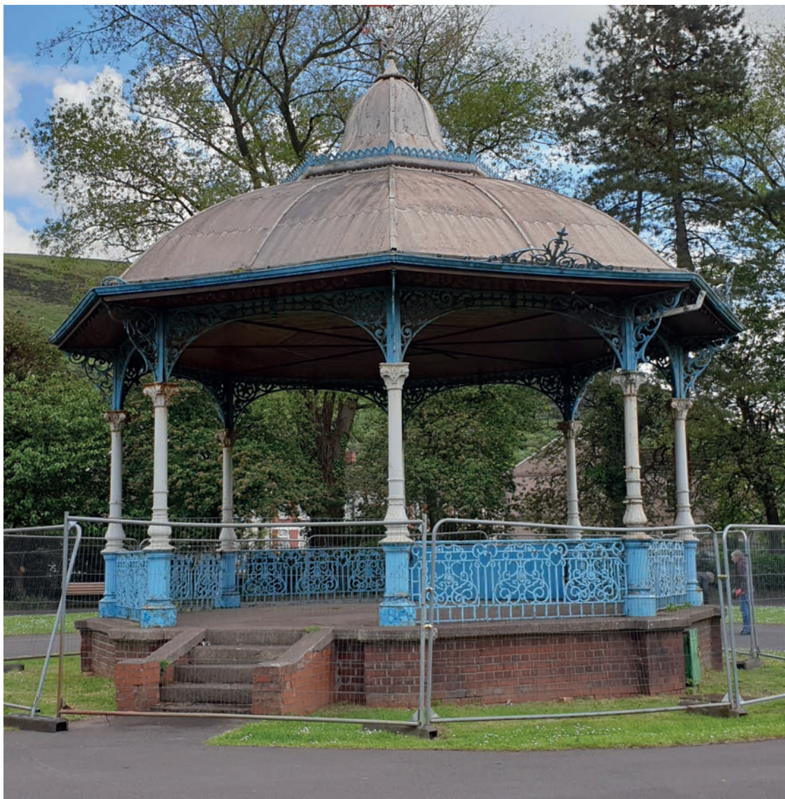
The Bandstand in Talbot Memorial Park in need for maintenance and repair.
