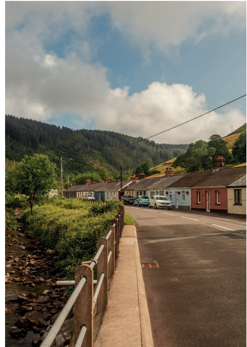
Gelli Houses, Cymmer (Grade II Listed Buildings).
