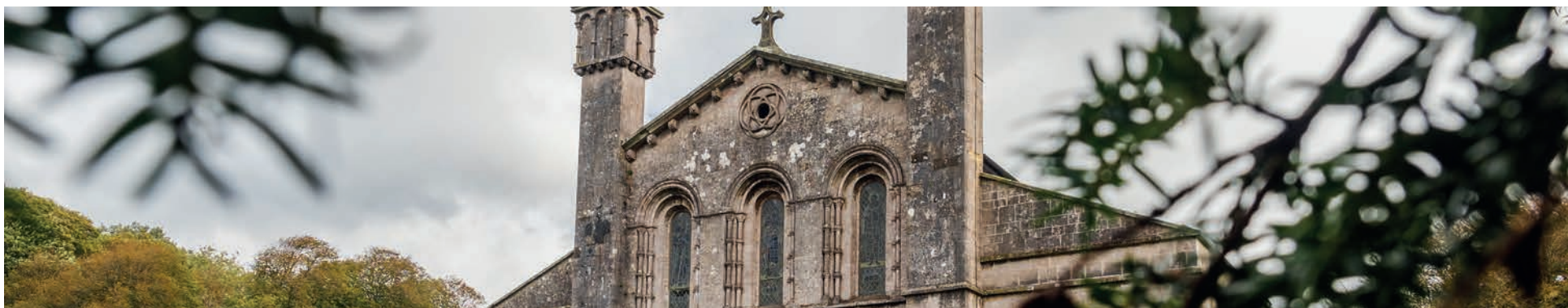
St Mary's Abbey Church, Margam (Grade I Listed Building).
